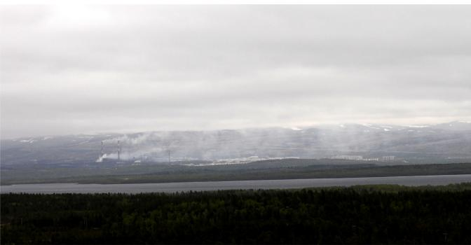
The Nickel smelter and the city of Nickel seen from Height 96 (Norway) 19 June 2008. Plumes from stacks as well as diffuse emissions from the buildings are clearly seen. Northerly wind brings the flue gas from the smelter towards the city. Hourly concentrations of SO<sub>2</sub> in the city of Nickel were about 1500 µg/m<sup>3</sup> when the photo was taken.
